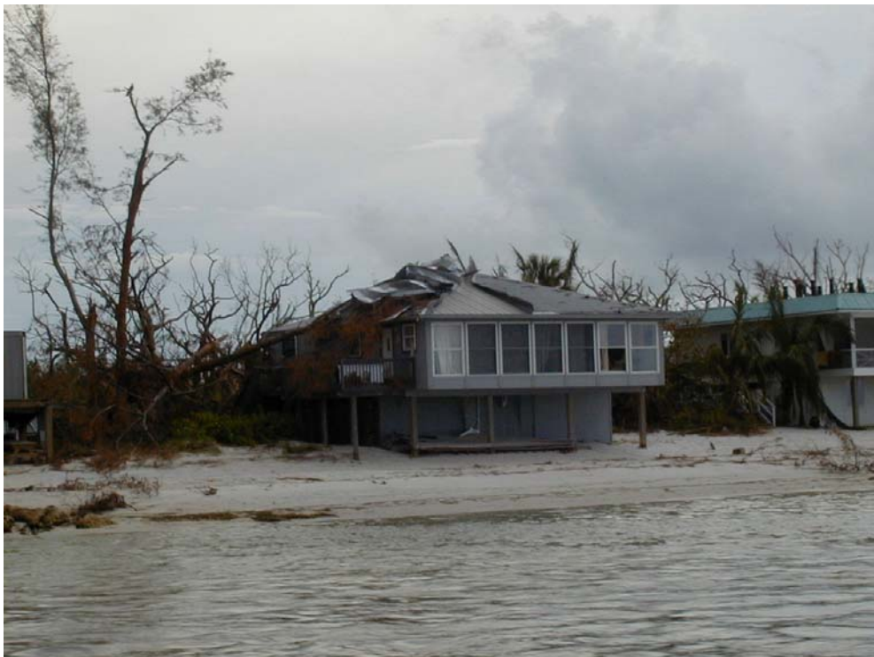
Photo 7. Typical structure damage to dwellings on North Captiva Island.
