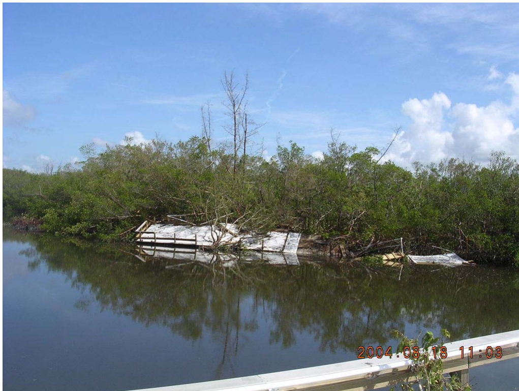
Photo 27. Pedestrian bridge destroyed at Lovers Key State Park (R217)
