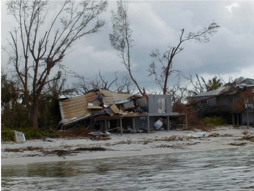
Photo 6. North Captiva Island dwelling destroyed.
