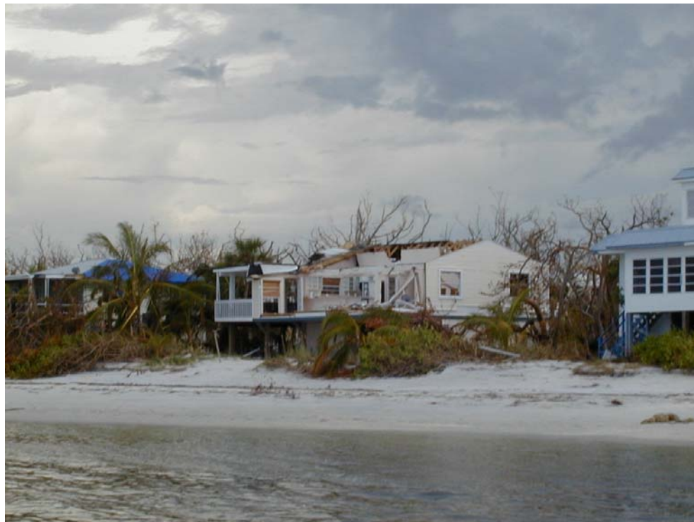
Photo 9. North Captiva Island dwelling destroyed
