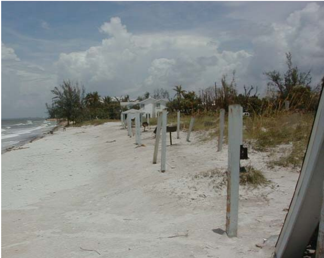
Photo 4. Gasparilla State Park shelters had roofs blown off.
