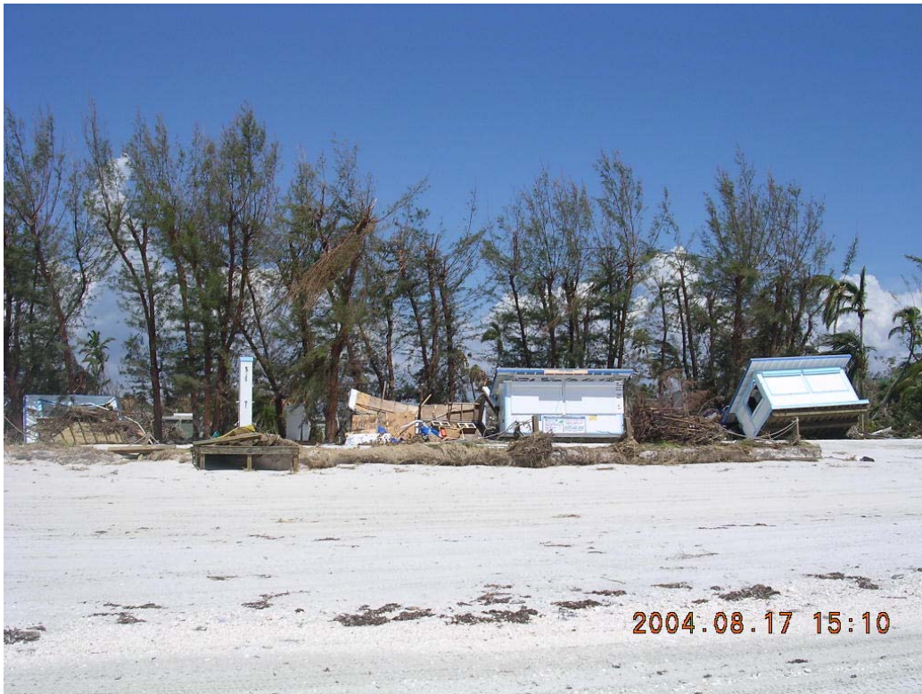
Photo 16. Typical flood damage, Captiva Island (R86)
