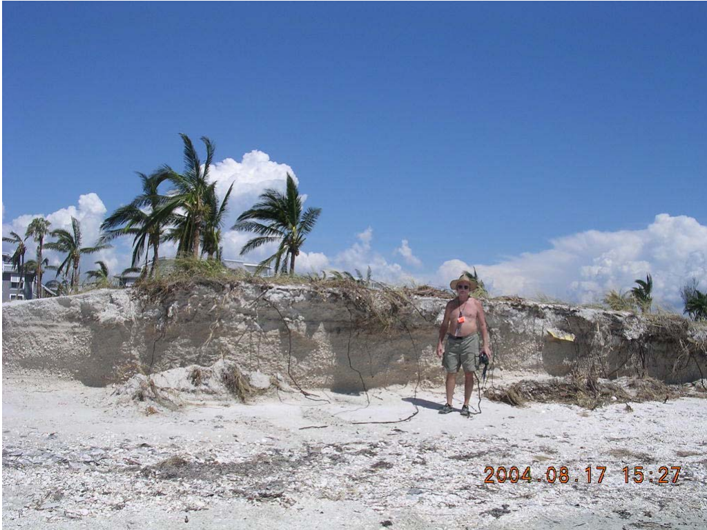
Photo 14. Condition IV erosion, Captiva Island (R84)
