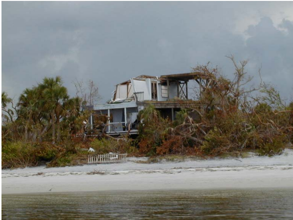
Photo 8. North Captiva Island dwelling destroyed.
