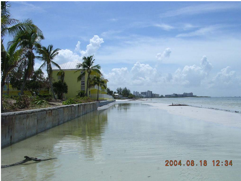
Photo 24. Scour trough with sandbar formation seaward of armoring (R195)
