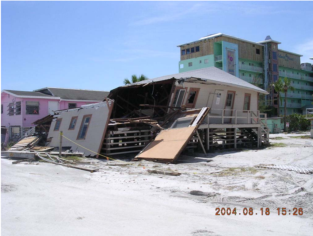
Photo 21. Estero Island dwelling destroyed (R183)
