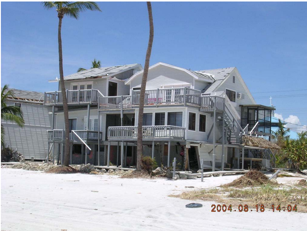
Photo 22. Estero Island dwelling with typical flood damage (R191)
