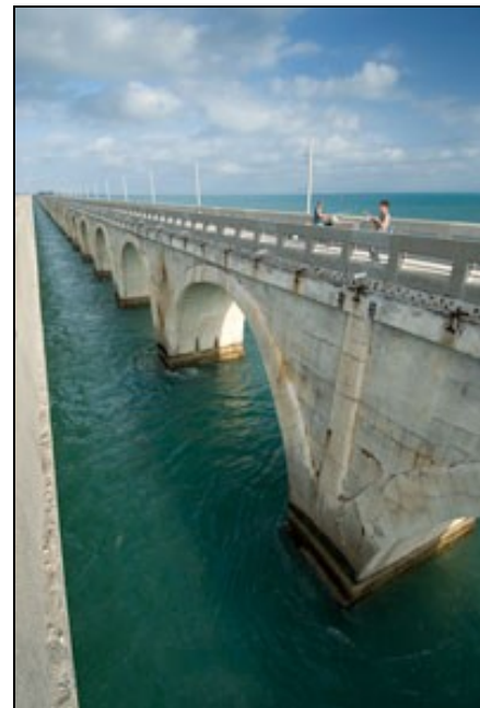
FKOHT Bridge Photo by John Moran
