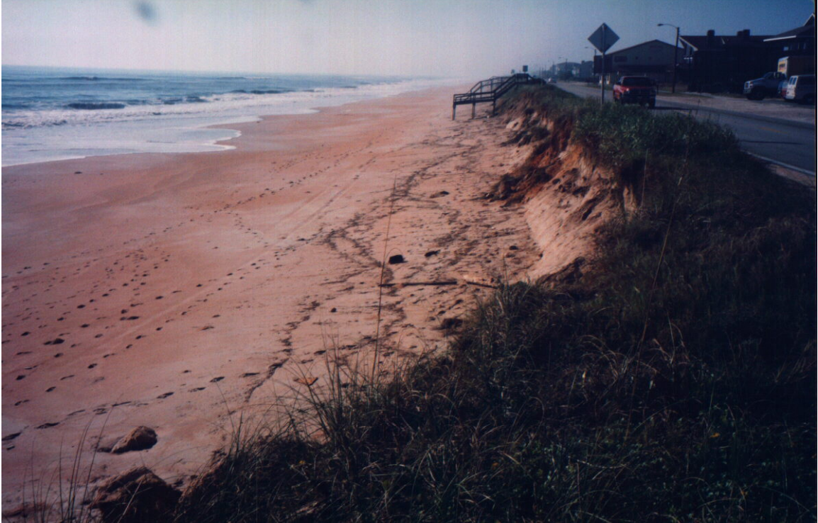
Photo 5. Floyd's erosion threatens State Road A1A in Flagler Beach south of 19 th Street.
