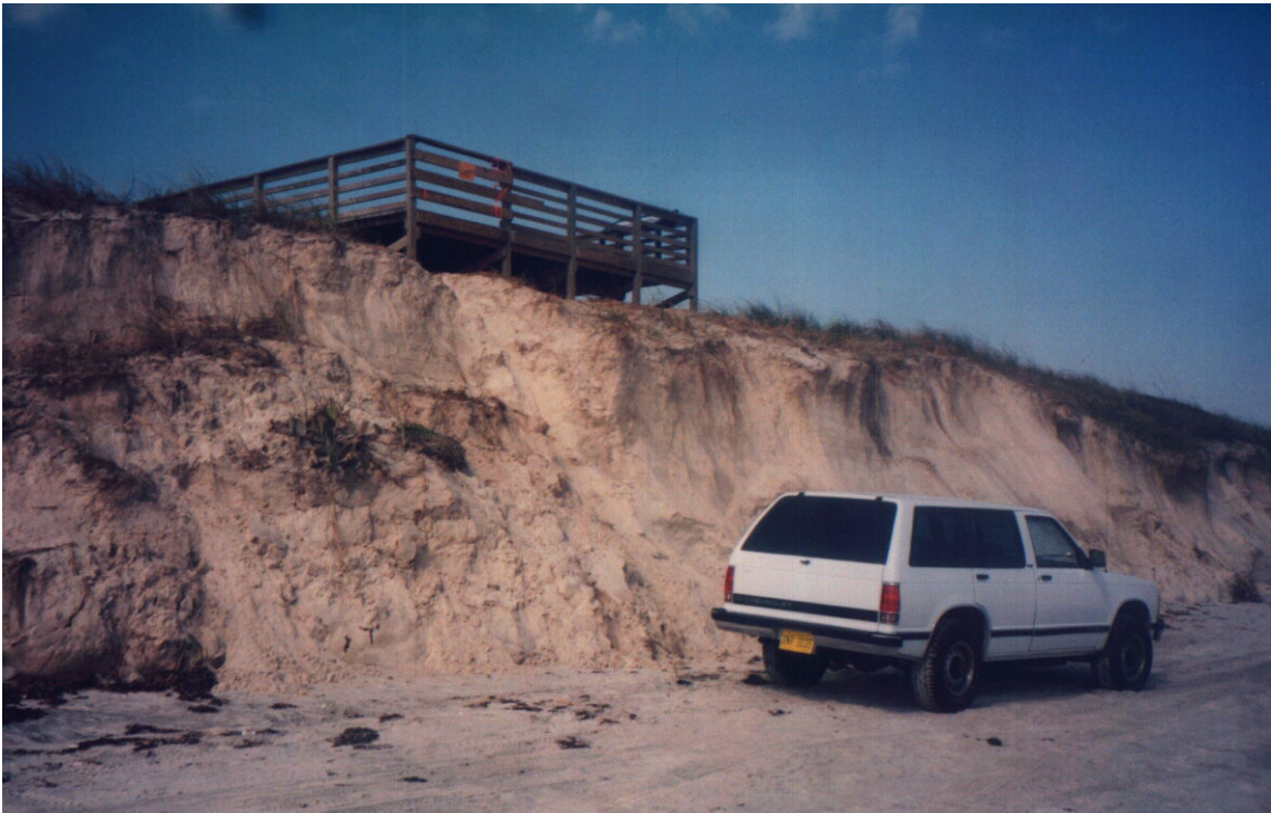
Photo 4. Ft. Matanzas continued dune erosion from Irene.
