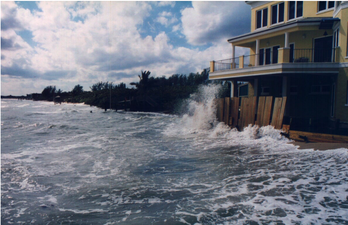
Photo 16. Severe erosion at Bathtub Reef, south Hutchinson Island (R34-R36).
