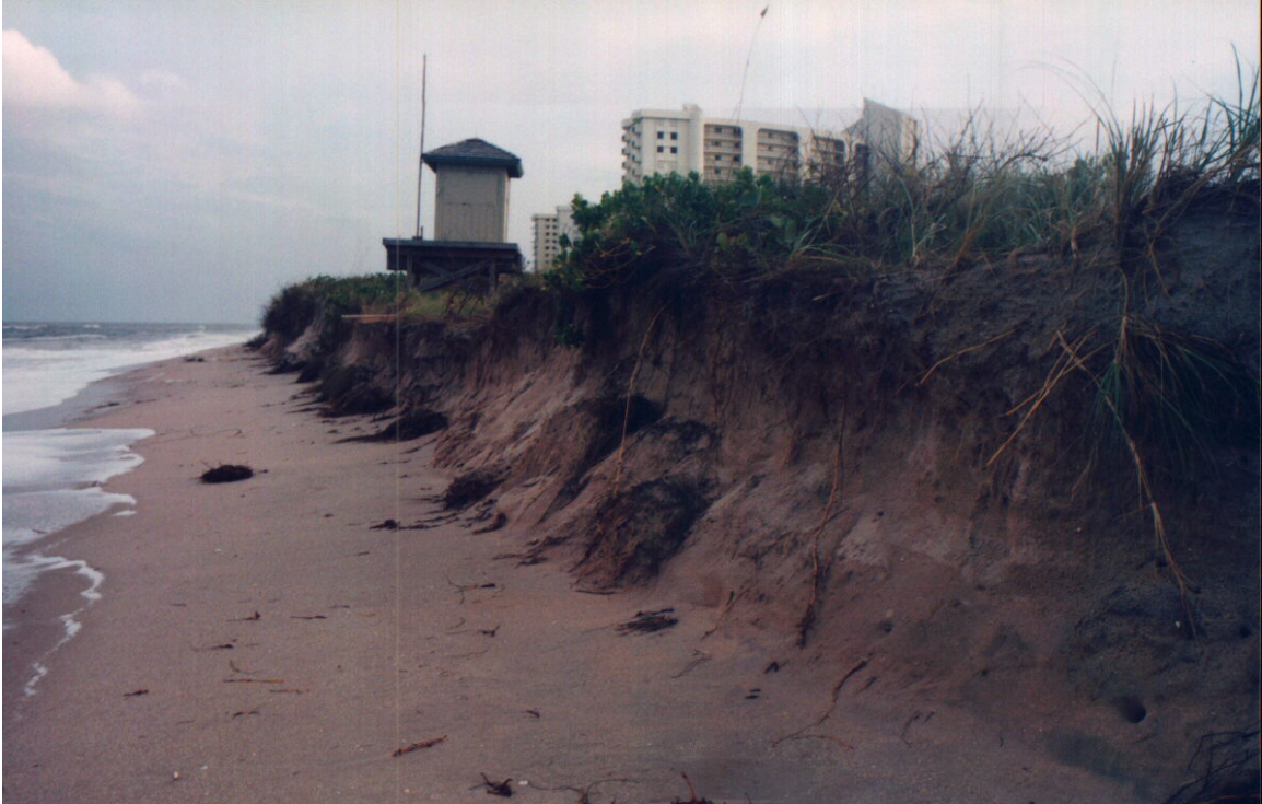
Photo 17. Severe beach and dune erosion south of Jupiter Inlet (R14-R15.5).
