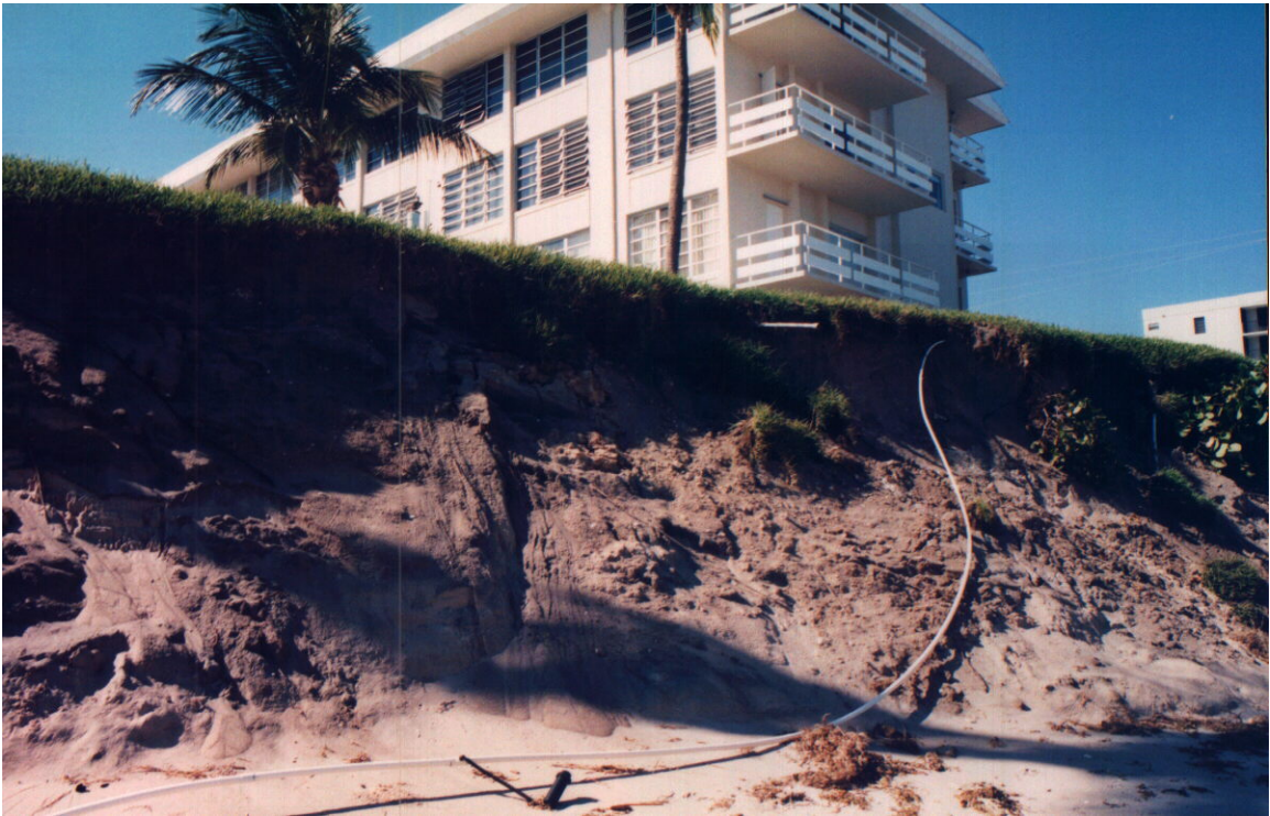
Photo 18. Severe dune erosion near Sea Lane in Gulfstream (R167-R168).
