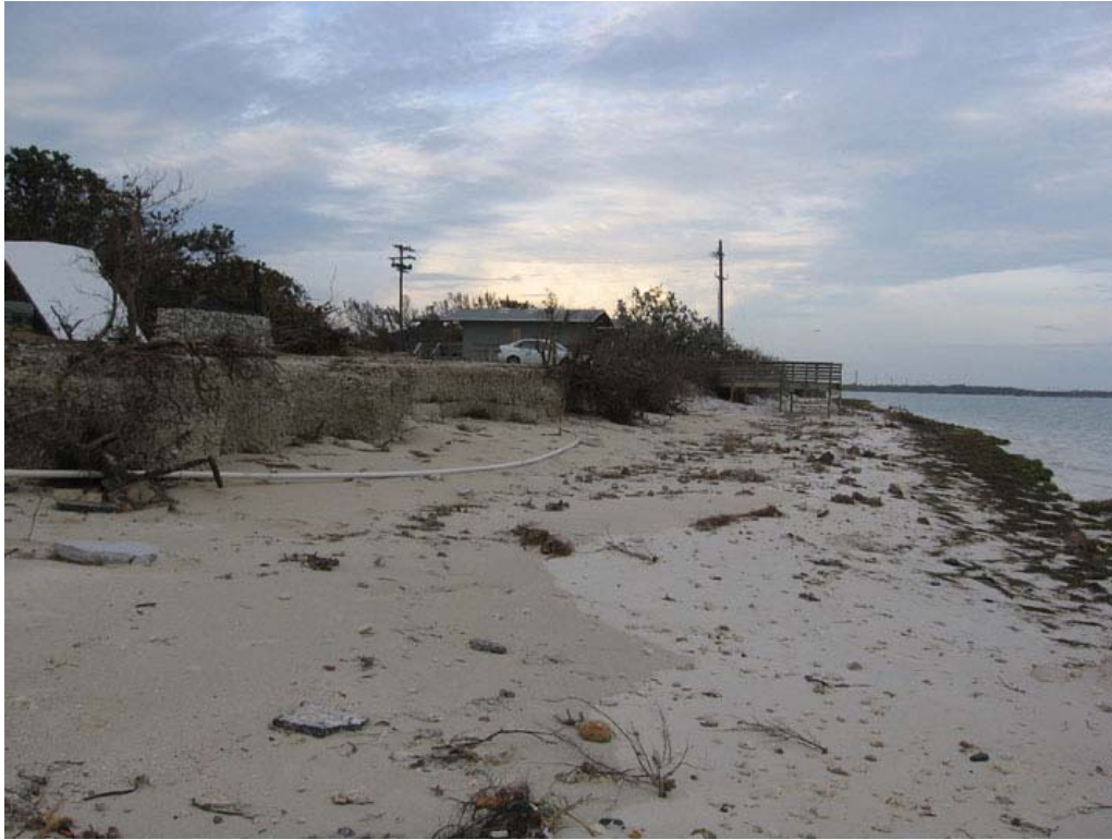
Photo 30. Severe erosion at Loggerhead Beach, Bahia Honda State Park.
