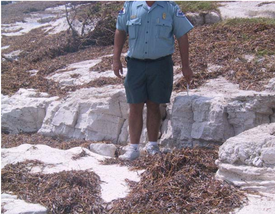
Photo 25. Significant erosion, Curry Hammocks State Park.
