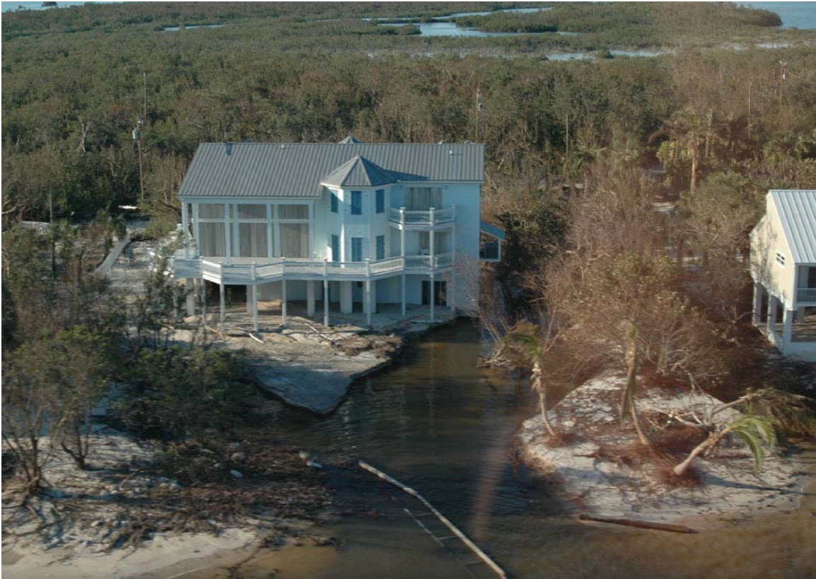
Photo 50. Imminently threatened dwelling, Sugarloaf Key.
