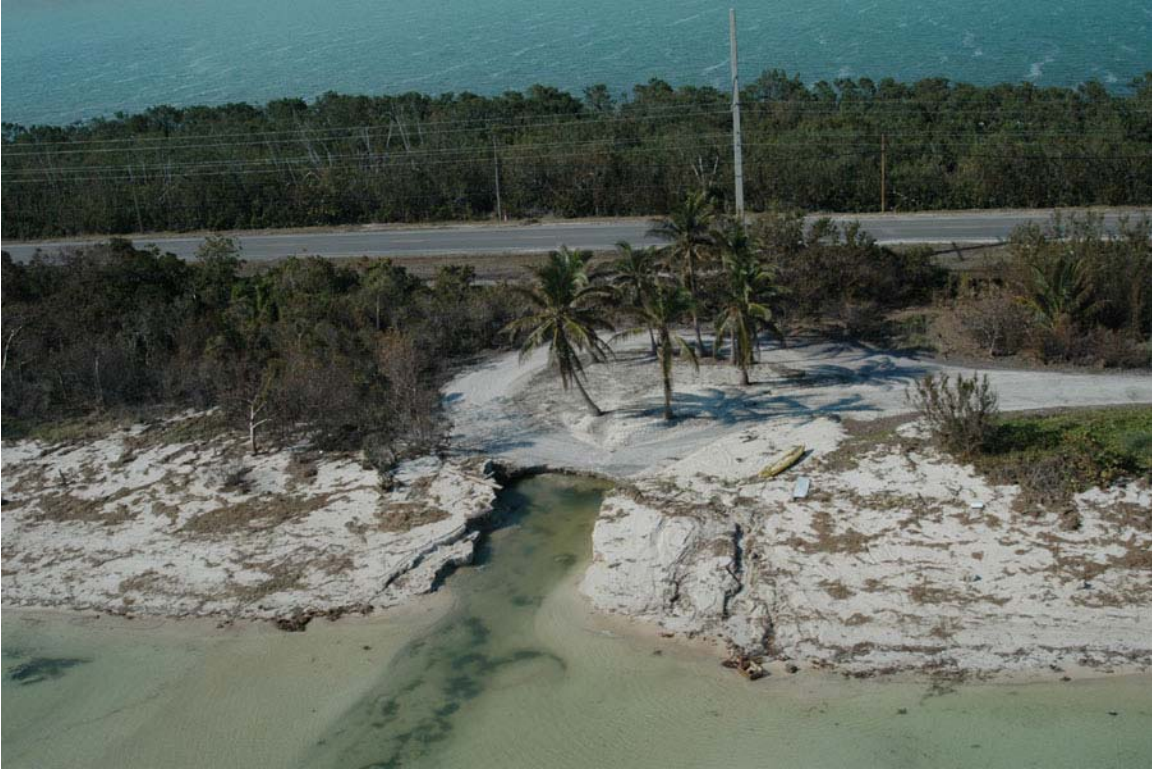
Photo 42. Storm surge discharge gully, Long Key State Park.
