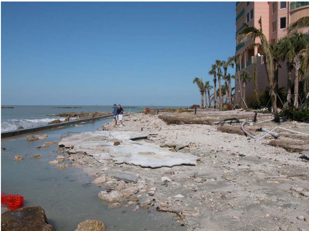
Photo 19. Seawall and revetment overtopped and damaged, south end of Marco Island.
