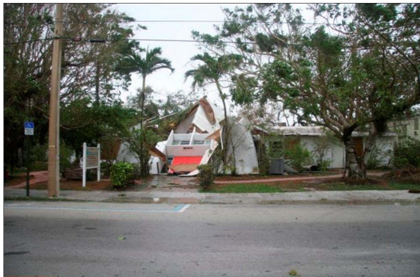
Photo 54. Key West wind damage.
