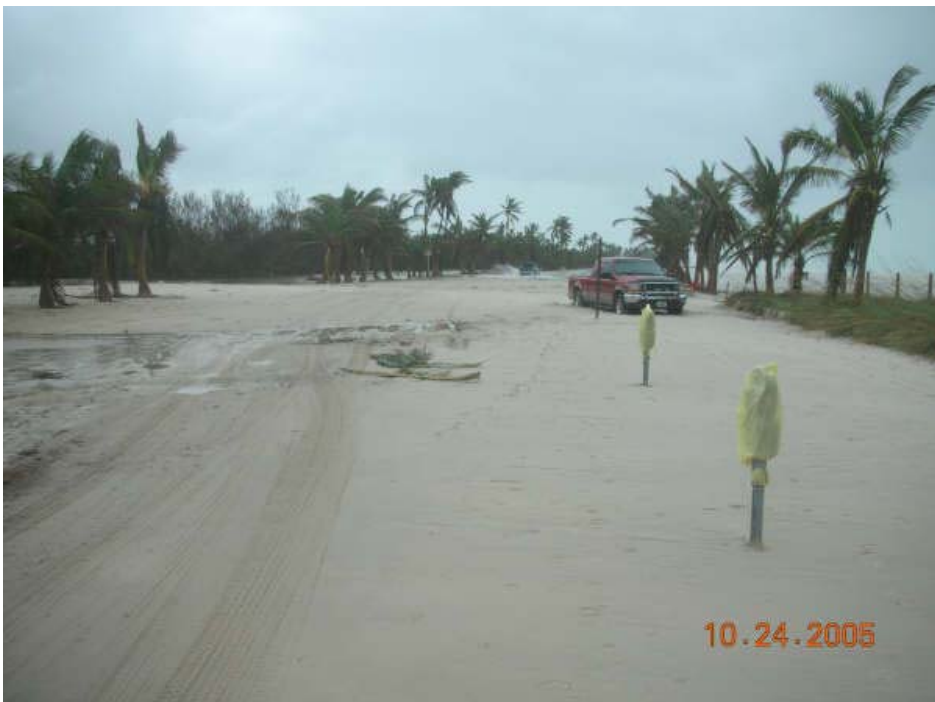
Photo 36. Overwash from Smathers Beach onto South Roosevelt Boulevard (Credit: City of Key West)
