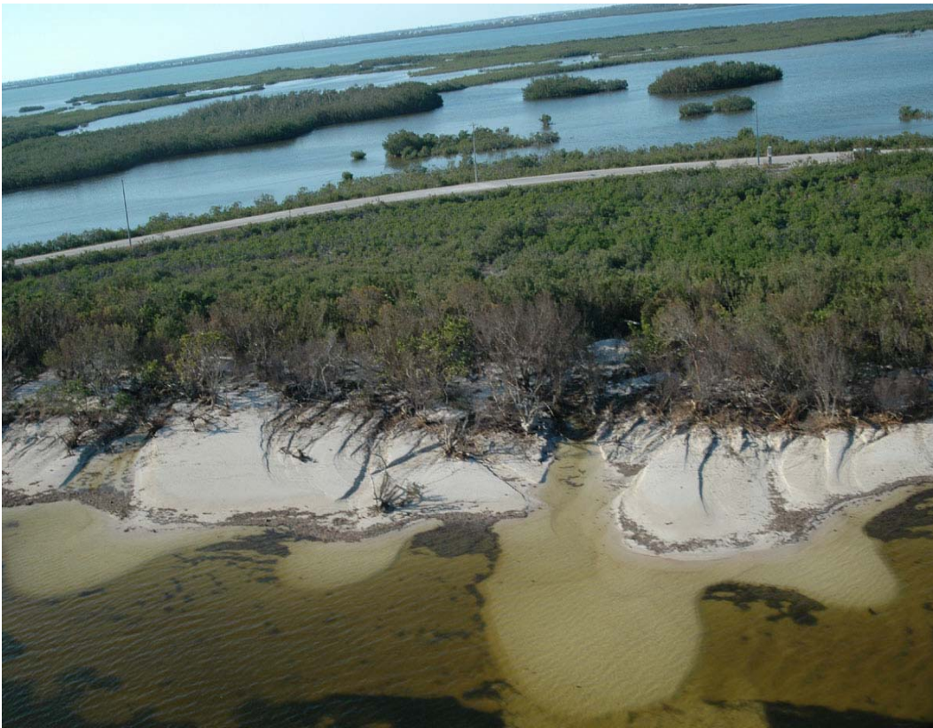
Photo 33. Storm surge discharge channels, Long Beach, Big Pine Key.
