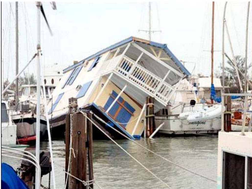
Photo 49. Damaged house boat, Garrison Bight.
